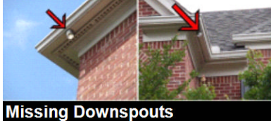
Missing Downspouts
